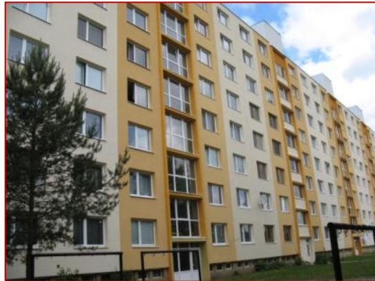
Modernisation of apartment buildings
