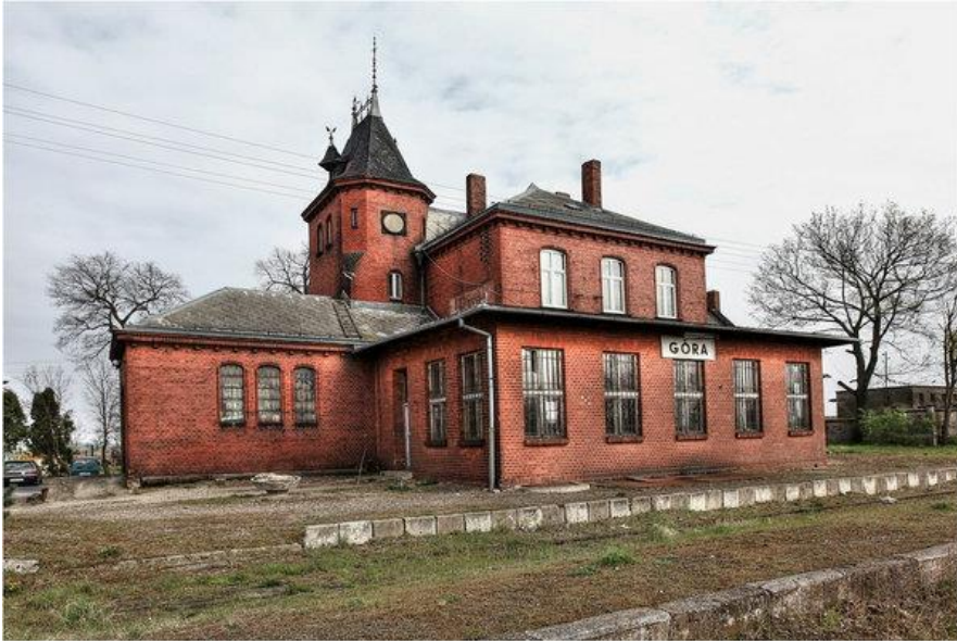
Railway station in Góra, building from 1898
